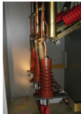
24kV Voltage Sensor installed in switchgear application
