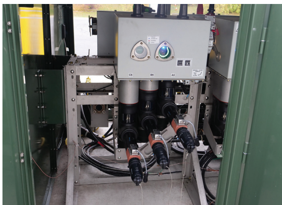
Underground platform with product installed (VS-27-UG)
