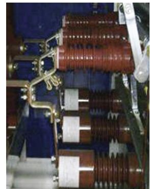
Voltage Sensor (VS-24-I – top) & Current Voltage Sensor (CVS-24-I – bottom) installed in switchgear application
