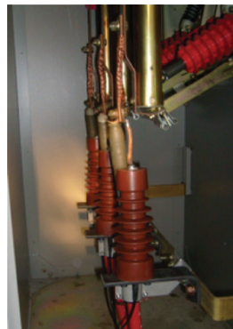
24kV Voltage Sensor installed in switchgear application
