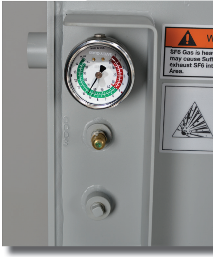
Pressure gauge and fill valve
