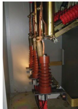
24kV Voltage Sensor installed in switchgear application
