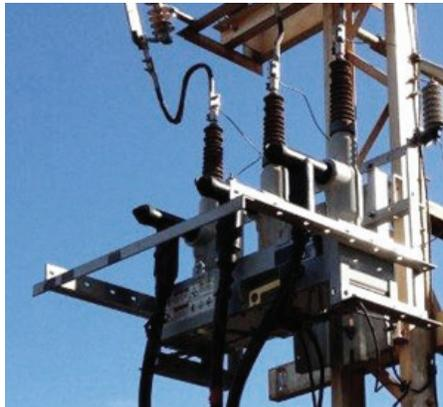
Figure 11: Elbow-Connected G&W Viper Reclosers
