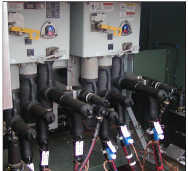
Image 2: Front/back access padmount switches incorporated two Trident-SR switches on both sides.
