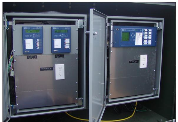
Image 3: SEL-751As and 451 were mounted in a common enclosure on the side of each switch.
