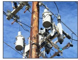
Viper-ST recloser with 6 VS, two control power PTs, and SEL-651R control
