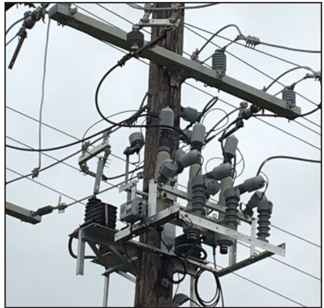
After: Accusense Retrofit Installed and in service
