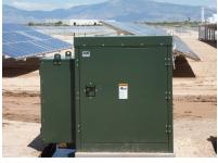
Padmounted Viper-S used in place of a circuit breaker in a solar generation intertie application
