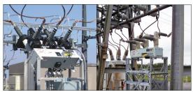
45° angle mounting for applications requiring the same load and line side connector height.
