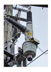
Maintenance-free - Encapsulation in solid dielectric epoxy provides a maintenance-free installation. Electronic equipment associated with the operation of the magnetic actuator is located in the control. The Kestrel control is able to monitor the battery status and contact wear to schedule for preventive end of life replacement.
