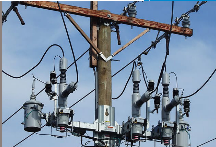
38kV Viper-ST recloser with center mount frame.
