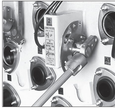
Three phase interrupter operating handle for manual three phase operation and reset.
