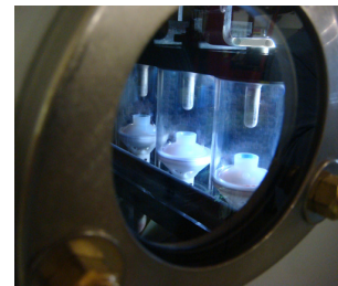
Three phase visible position of contacts.
