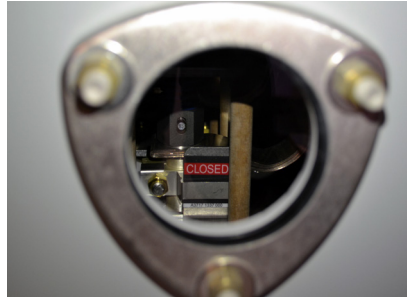
Position indicators provide contact position indication through viewing windows.
