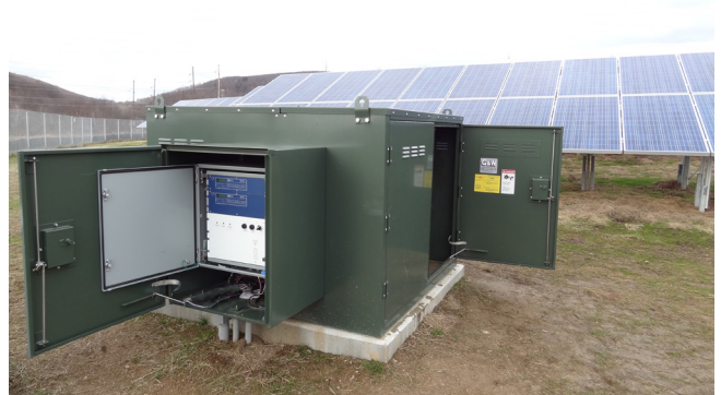
Padmount switch with SEL controls.
