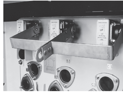
Interrupter operating handles for manual single phase (left) or three phase (right) operation and reset. Motor actuators can be added to three phase for remote operation.
