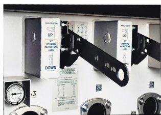
Single phase interrupter operating handles.
