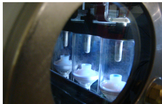
Load break switch visible break.
