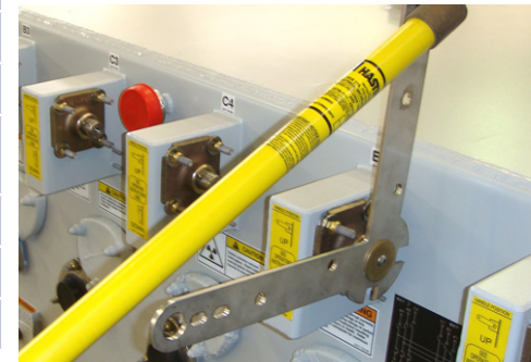
Interrupter with dual operating handle.
