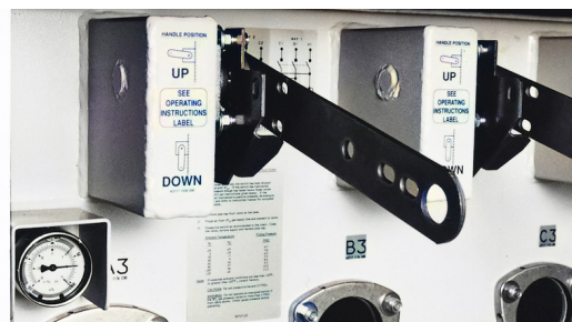
Single phase interrupter operating handles.
