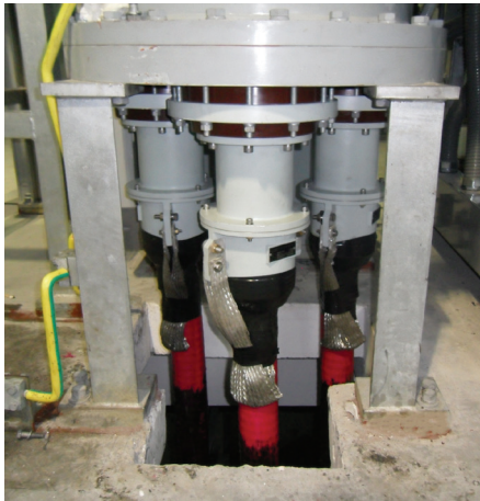
SSC140-SF terminations installed in a GIS.
