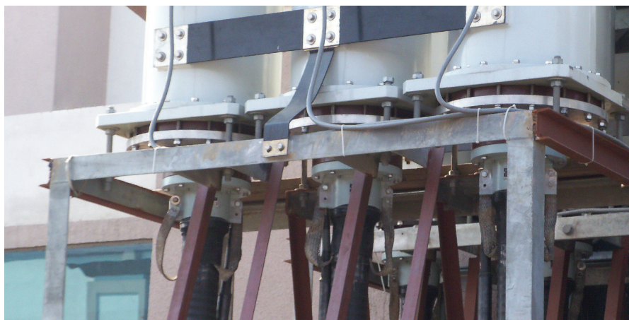
PATR140-SF terminations installed in a GIS.
