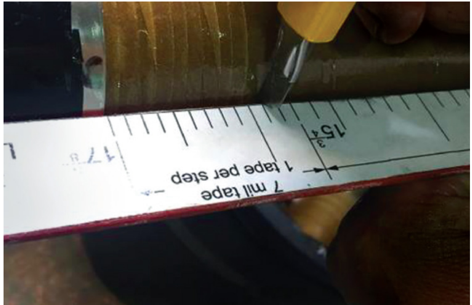
Template for insulation stepping is designed for specific cable and provided in the joint kit.
