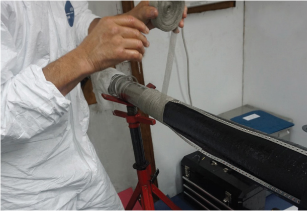
Application of the tinned copper braid over the ground electrode of the joint.
