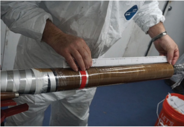
Template for building the stress cone slope is designed per specific cable and provided with the kit.
