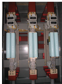
CLiP used in a large offshore deepwater oil platform
