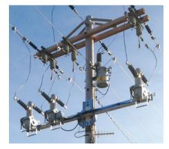
Figure 9: G&W Viper Recloser With Z-Shaped Modules and Extended Phase Spacing
