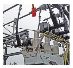
Figure 11: Elbow-Connected G&W Viper Reclosers
