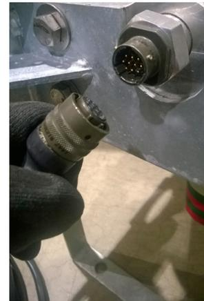
*A standard hardwired control cable is provided on the Viper-SP module end. As an option, a connectorized module can be provided.*
