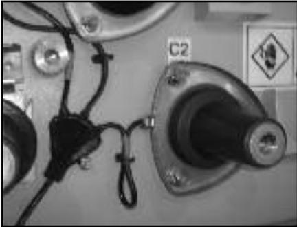
The VS bushing system utilizes a capacitively coupled screen which is embedded within the epoxy bushing. The low energy output of the screen is amplified by integral circuitry, resulting in a 0-120 VAC analog output suitable for direct connection to any relay, IED or RTU. The circuitry incorporates built-in calibration and temperature compensation which improve accuracy.
